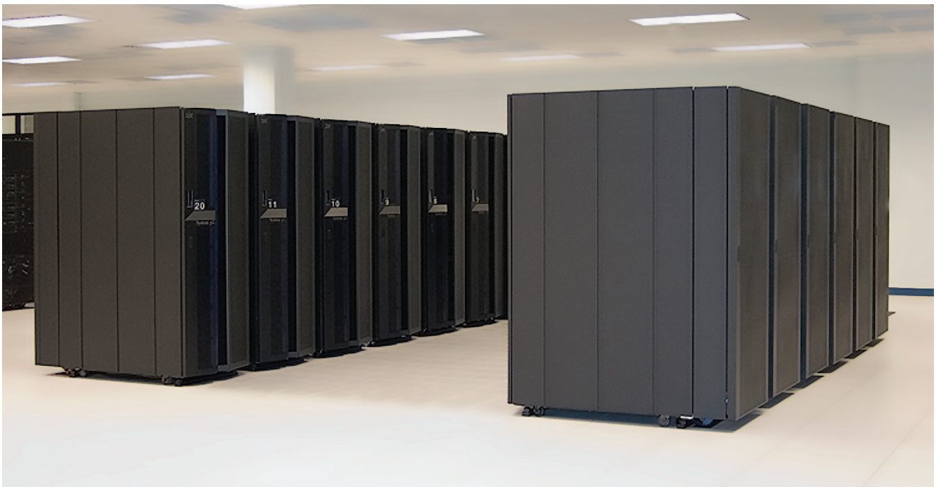
TI-06 IBM Power5+ Systems on the NAVO MSRC Computer Floor.
